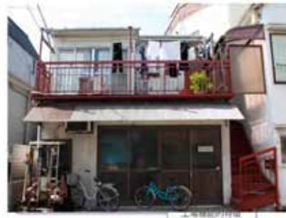
Figure: images of “Live-Fab. Building”
